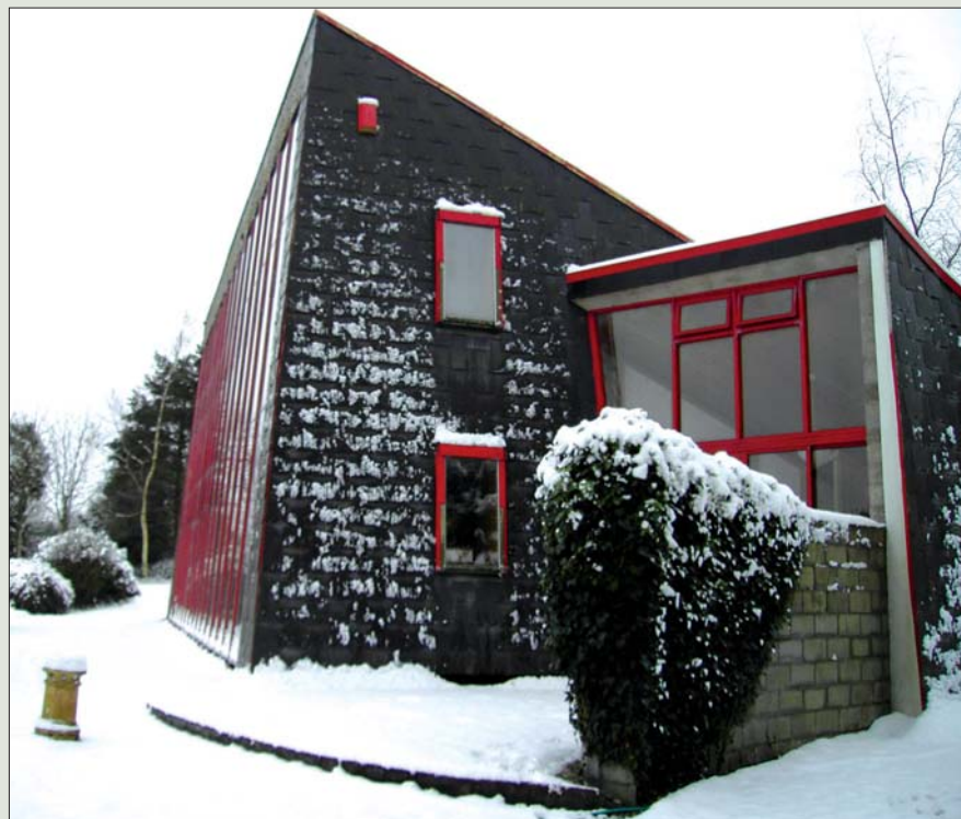
(above) Ireland's first example of a passive solar house in Garristown, County Dublin, featured a solar wall of some 110m 2 ; (below) the Knocklyon solar house featured a solar heating and ventilation system; (opposite, top) a clay / straw passive house in Tattendorf, Austria; (opposite, bottom) a NuTech designed passive solar house built with KTF's innovative timber frame system
